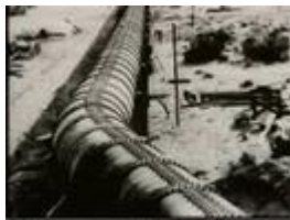
Construction of the Owens Valley Project
